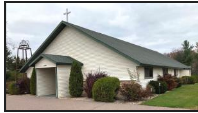
ST. MICHAEL CHAPEL- Chute Pond
